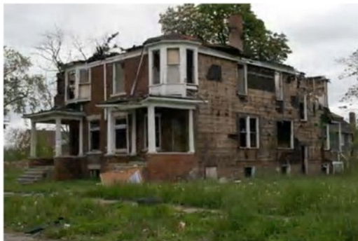
Abandoned house on Detroit's east side
